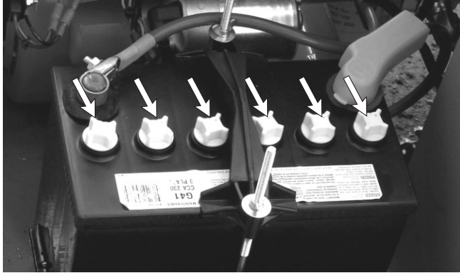
Figure 9.6 - Battery Fluid Level
