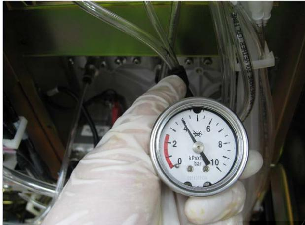
8. Turn on the AIR pipeline supply and record the reading on the test pressure gauge. If the difference between this reading and the reading on the AIR pipeline pressure gauge is more than 0.1 MPa (1 bar), it indicates that the AIR pipeline pressure gauge is damaged. Handle this problem as described in the troubleshooting table.
