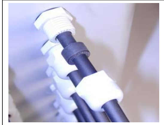
Figure 11. Connecting Cables to Enclosure
